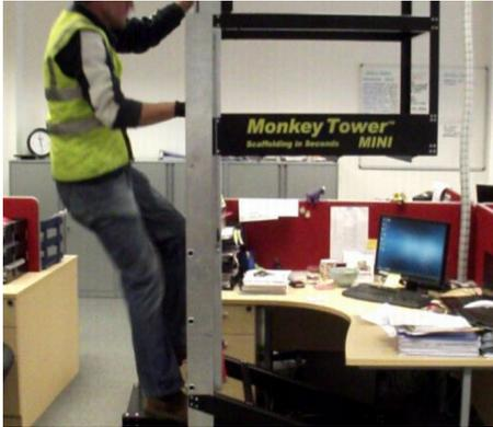
**▲ DANGER** *Do not extend the height of the platform by climbing on the guardrails or by using ladders, boxes etc.*
